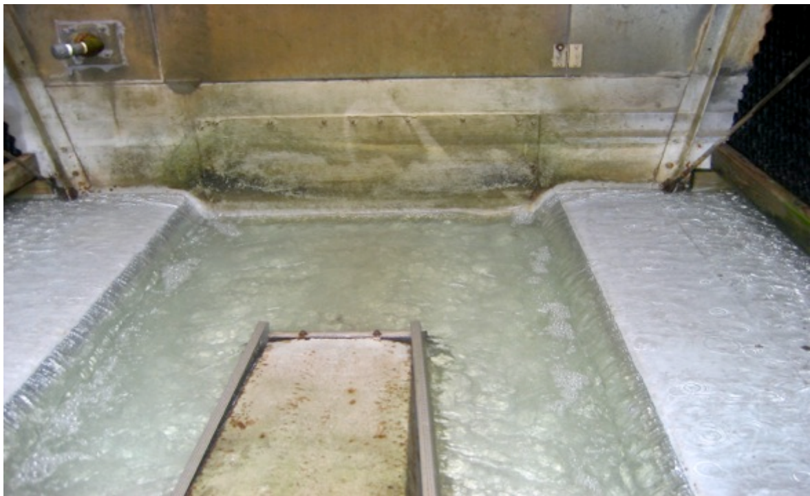
Water after two years treatment with ProMoss™ Note clarity, absence of foam and organic contamination
